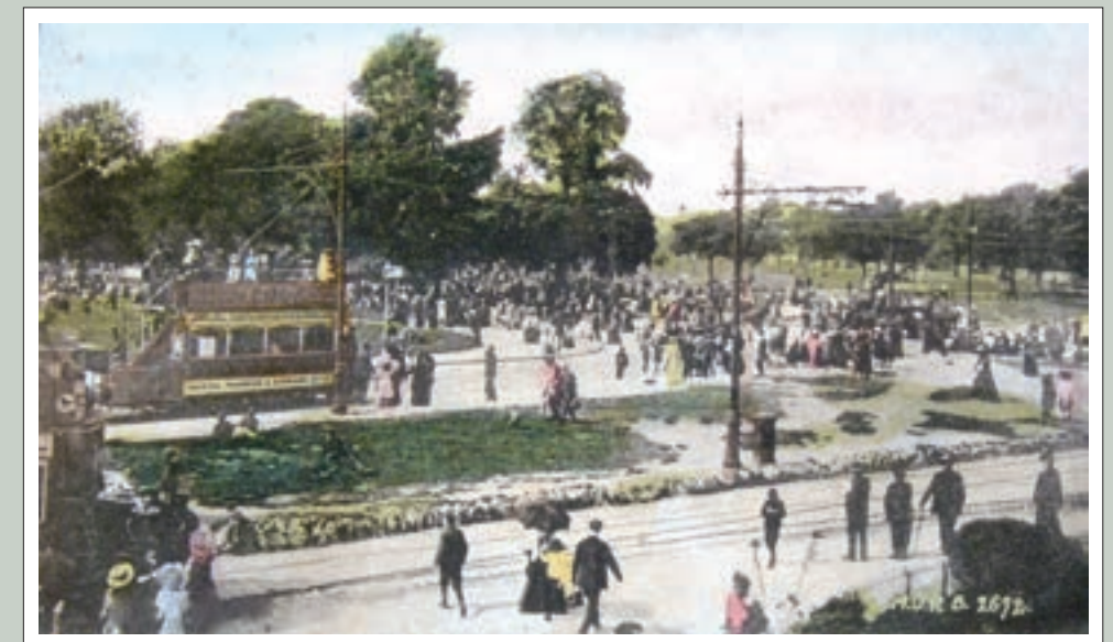
Tram terminus on the Downs at the junction with Stoke Road, c.1905; postcard (BRO43207.9.35.133)
